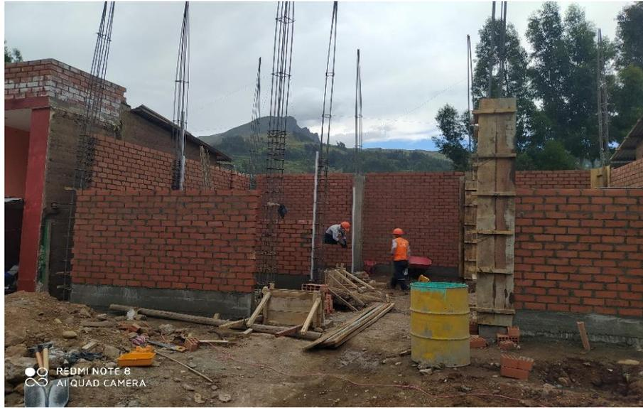
FOTO N°4: SE OBSERVA LA COLUMNA DESENCOFRADA
